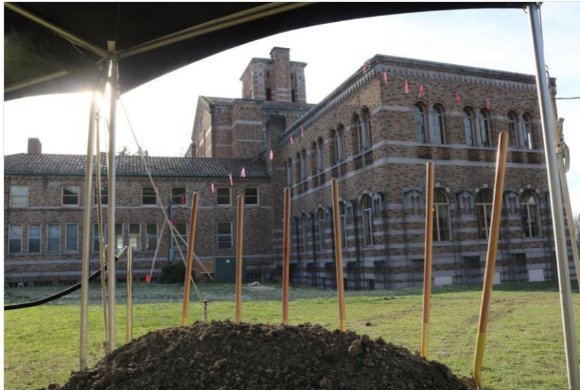
Golden shovels were available for photo opportunities at the ceremonial groundbreaking for the Lodge at Saint Edward Park on Dec. 7. Katie Metzger/staff photo
